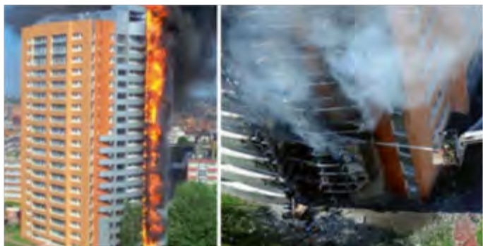
Fig. 5.12 Mermoz Tower during and after façade fire [45]
